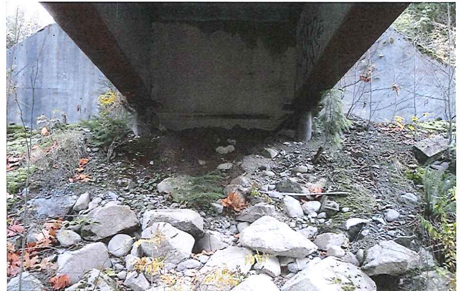
CK2095 Abutment Left Bank
