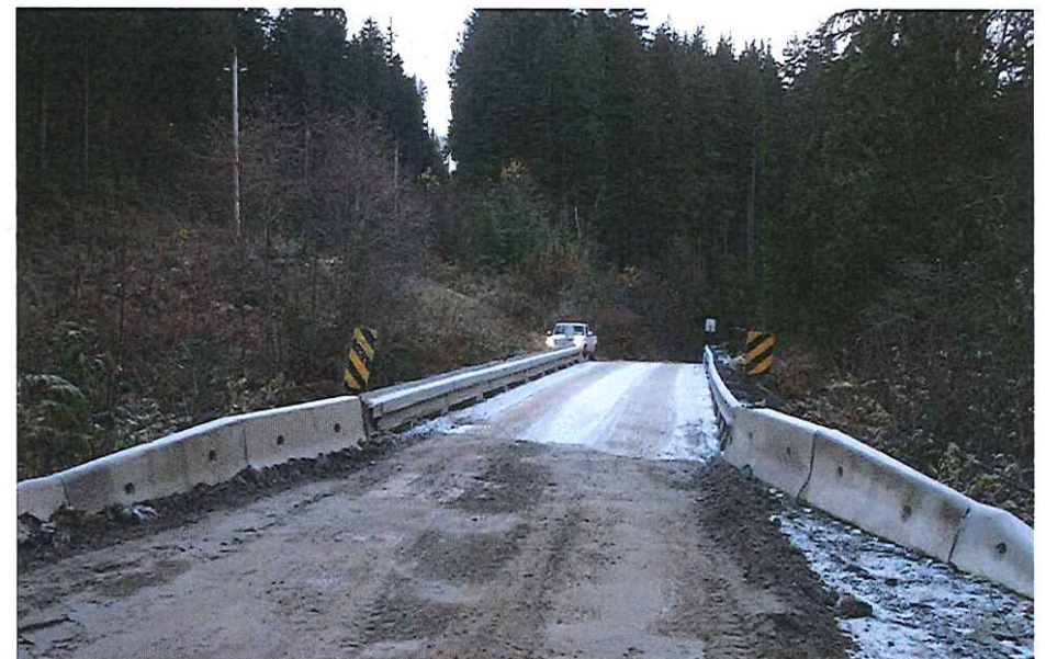
CK2095 Approach Right Bank
