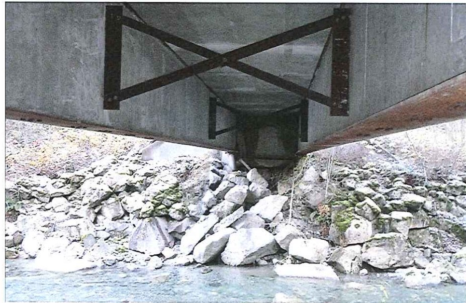
CK2095 Abutment Right Bank
